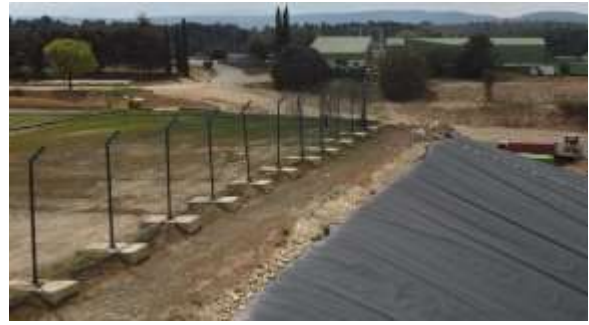
Filets de protection anti-envols
